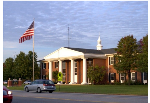
Lathrup Village City Hall
